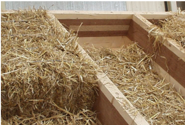
Figure 2. Wooden panel insulated with straw bales
